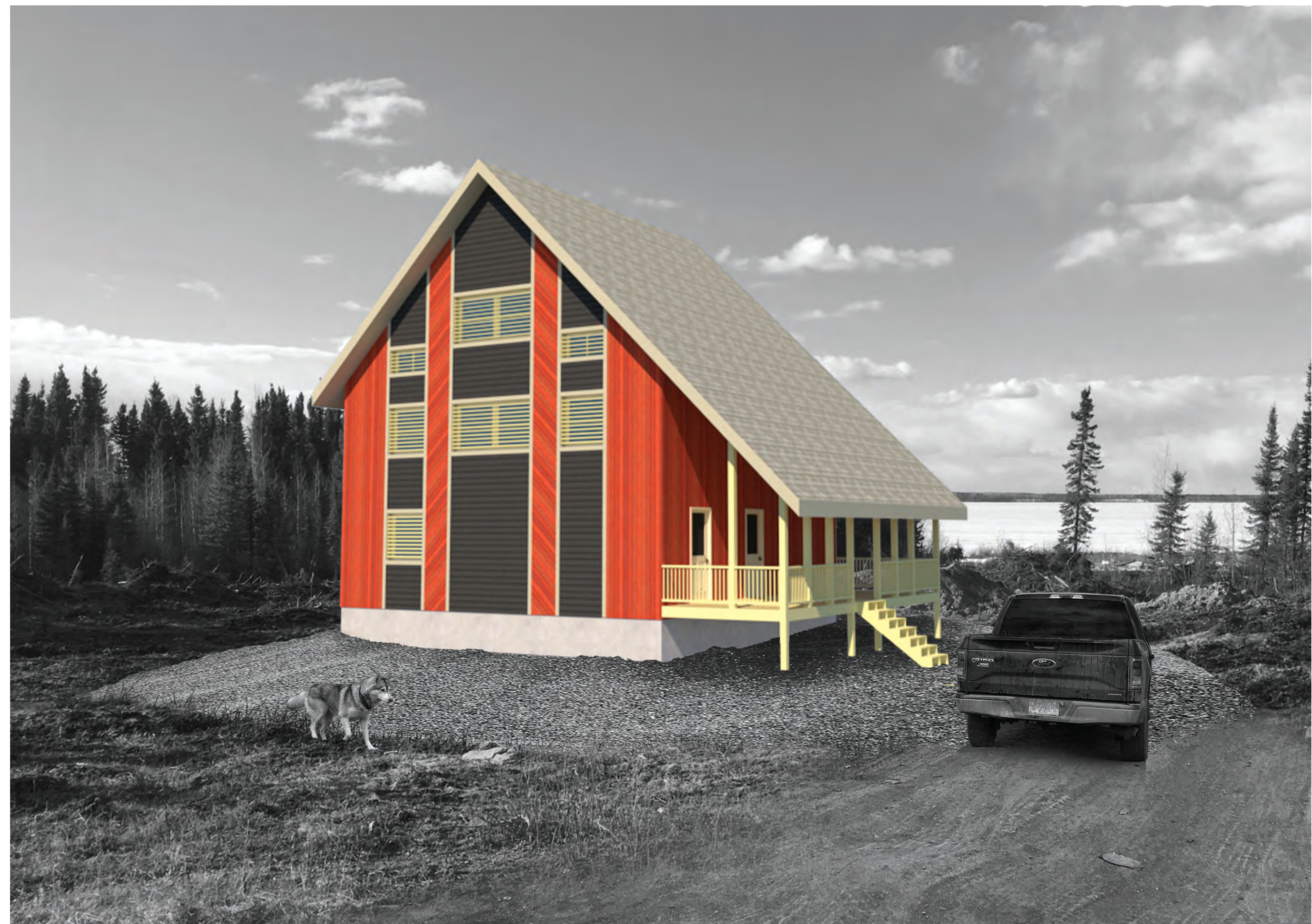
2.5 STOREY HOUSE RENDER - CRAWLSPACE ON GRANULAR FILL
